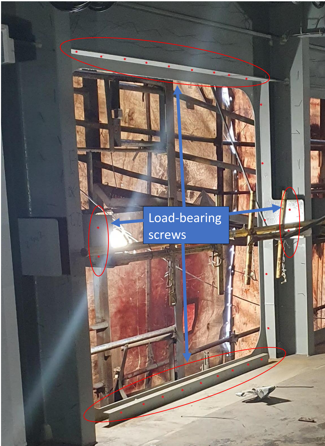
Figure 9-3 Screws fastening. The red dots show the location of the screws. The load-bearing screws are highlighted.
