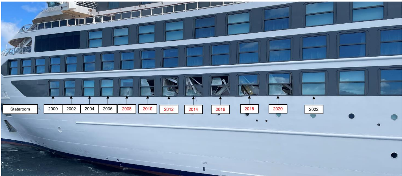
Figure 16: Staterooms where the windows were damaged indicated in red. Photo: NSIA
