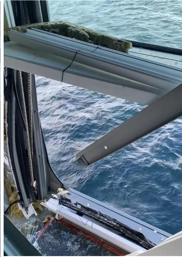
Figure 29: Window frame in stateroom 2018. Photo: NSIA
