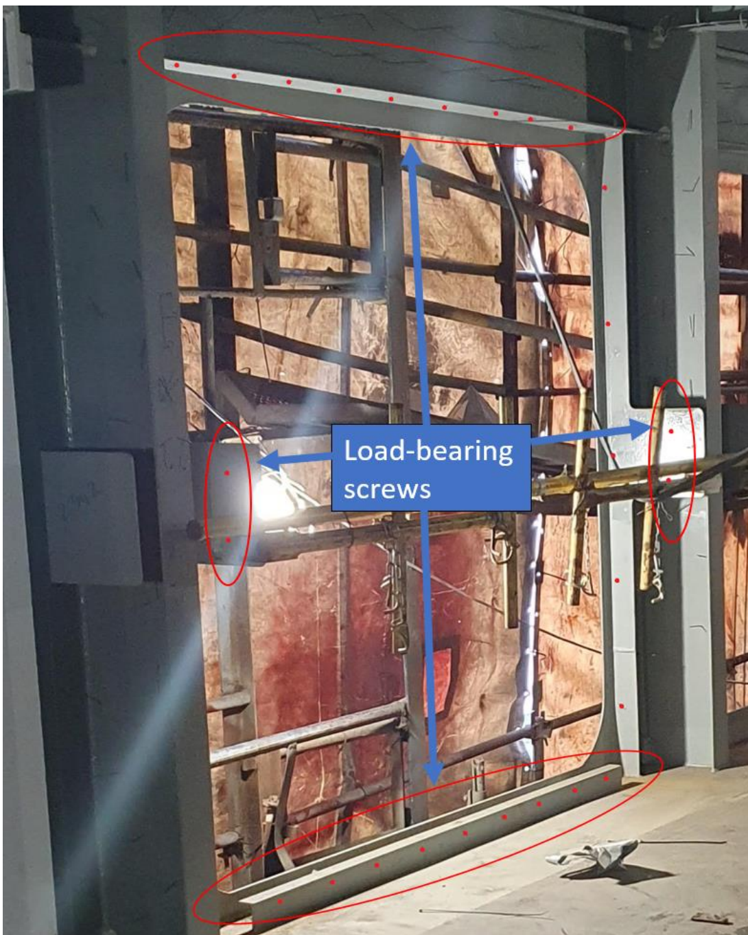
Figure 73: Screws fastening. The red dots show the location of the screws. The load-bearing screws are highlighted. Photo: Window supplier / modified by the consultant
