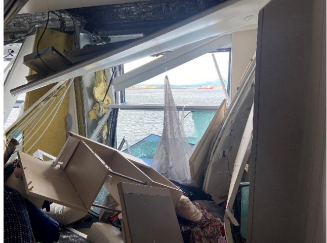
Figure 33: Damage in stateroom 2012. Photo: NSIA
