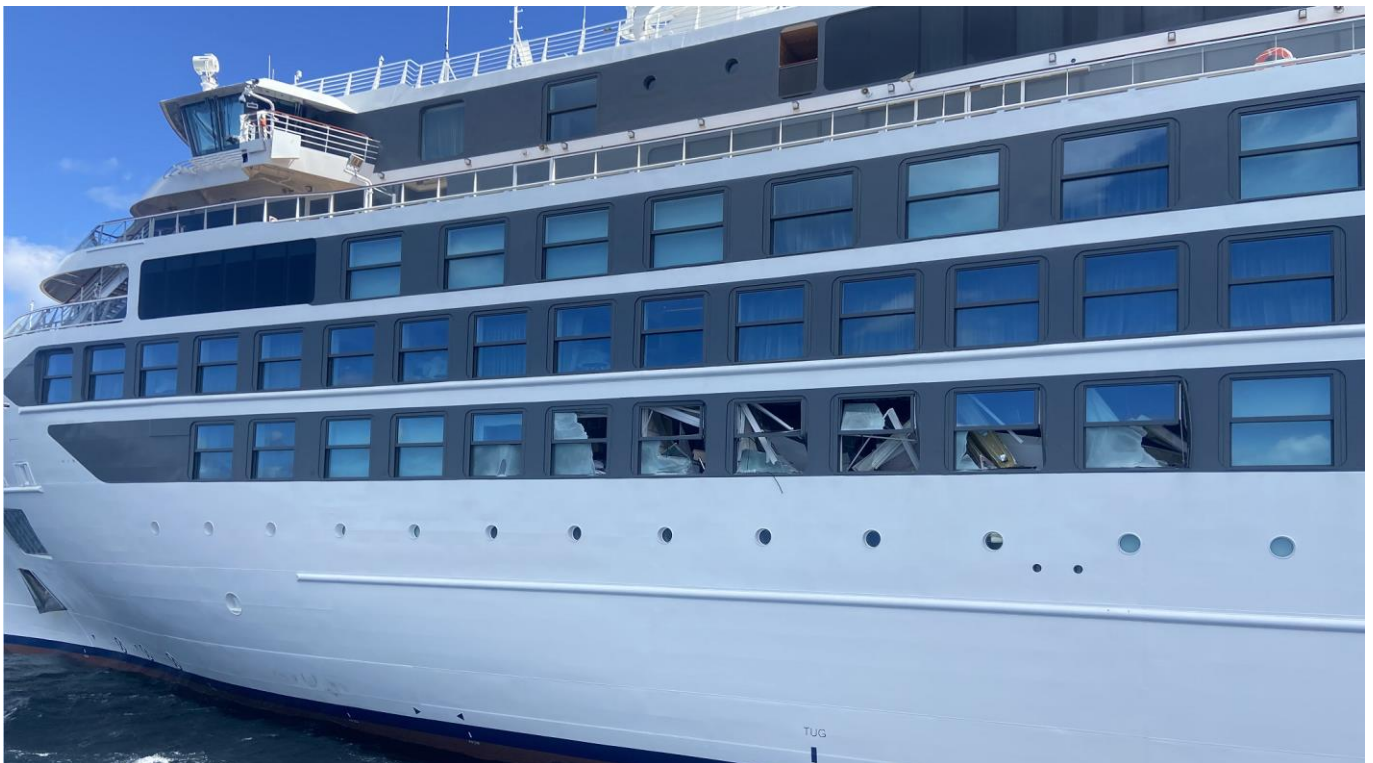
Figure 6-2 Photo of damage to the port side of 'Viking Polaris', deck 2, November 2022
