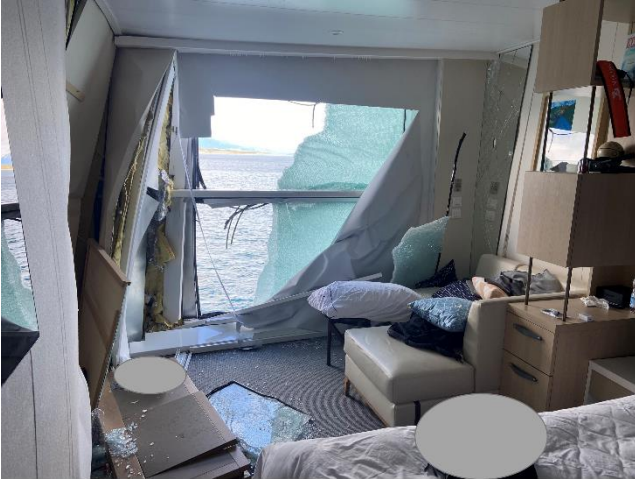
Figure 32: Damage in stateroom 2010. Photo: NSIA
