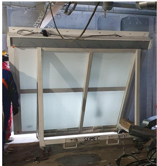
Figure 62: Window ready to be installed. Note the bolt holes on top of the frame and the horizontal stiffener in the middle of the window. Photo: Shipyard
